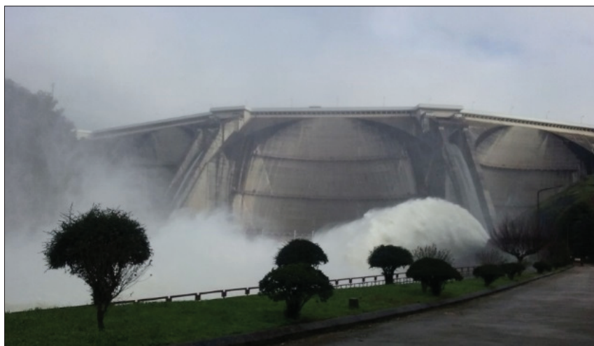
Fot. 1 - Pormenor de descarga da Barragem Aguieira (Fonte: CDOS de Coimbra, 2019). Photo 1 - Detail of the Aguieira Dam discharge (Source: CDOS Coimbra, 2019).
