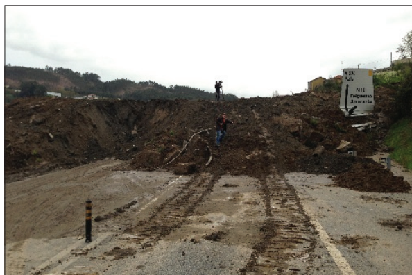
Photo 2 - Affected houses, where you can see the piling on which they were built, and the volume of debris from the landslide that accumulated on the Guimarães-Fafe road (Photography of Câmara Municipal de Guimarães, taken on 03/04/2013).
